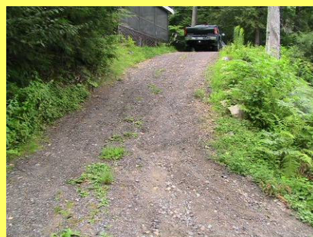
Before — Stormwater washes sediment down steep driveway into lake.
