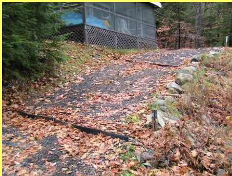
After — The driveway was resurfaced and graded, and “rubber razors” were installed to direct water off the driveway and into vegetation.
