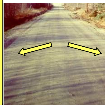
Crown —Grade the road so that water runs off the sides. Remove sand and grader berms from the edges of the road.
