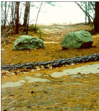
Waterbars —Place timbers or log "speed bumps" across paths to slow runoff and trap soil.
