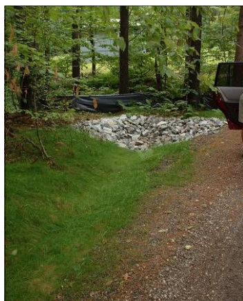
Ponding Areas —Create small ponding areas to trap sediment and infiltrate driveway runoff.
