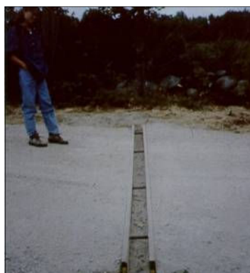
Open Top Culverts —Direct water off the road or driveway with open top culverts.
